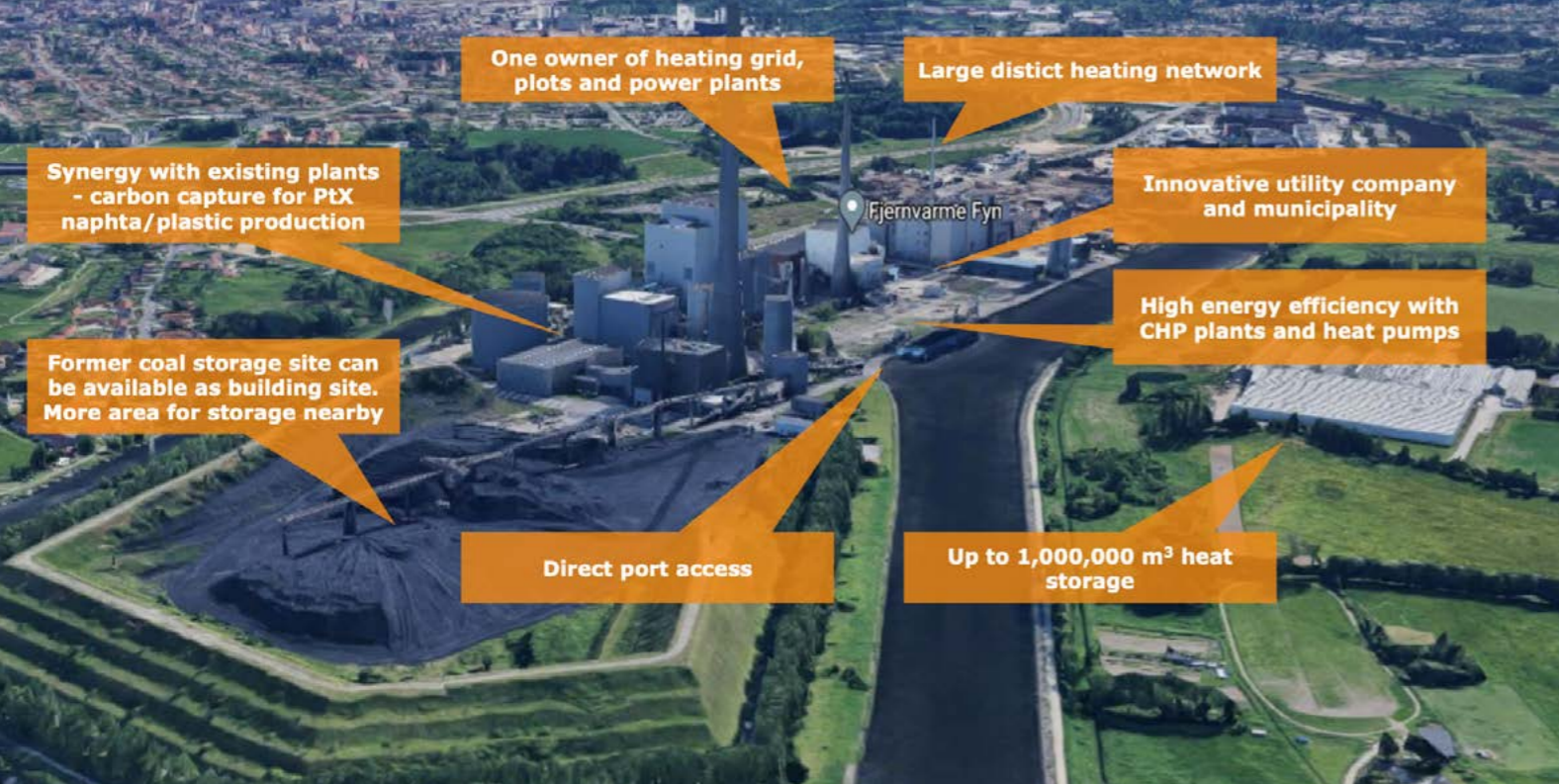
Figure 14. The power plant site in Odense is one of the possible locations for a PtX plant. The aerial photo illustrates how close to each other PtX and district heating can be located on the existing power plant sites. Source: Fjernvarme Fyn
